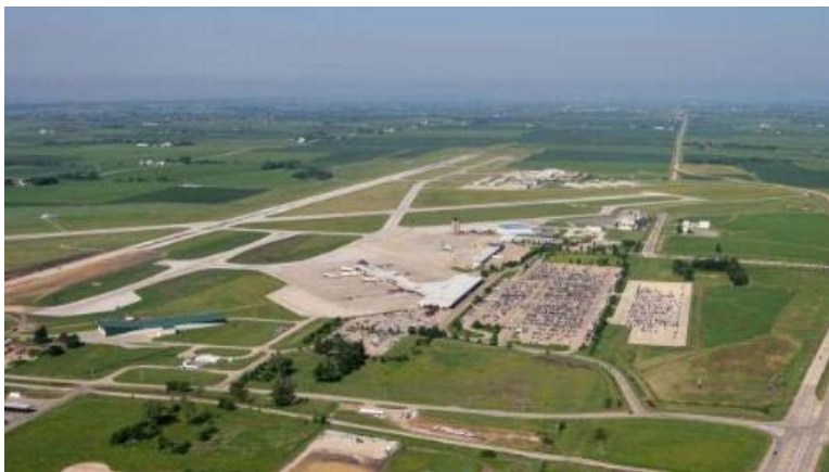
The Eastern Iowa Airport near Cedar Rapids, Iowa, aerial photo looking west with runway construction work on left side and Wright Brothers Boulevard lower right side, 6/23/2006.
